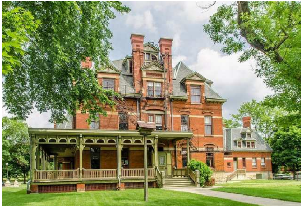
HOTEL FLORENCE : FLOOR TO FLOOR HEIGHT OF FIRST FLOOR APPEARS TO BE 11'-4". FLOOR TO FLOOR DIMENSION IS REDUCED APPROX. 8" ON SECOND AND THIRD FLOORS.
